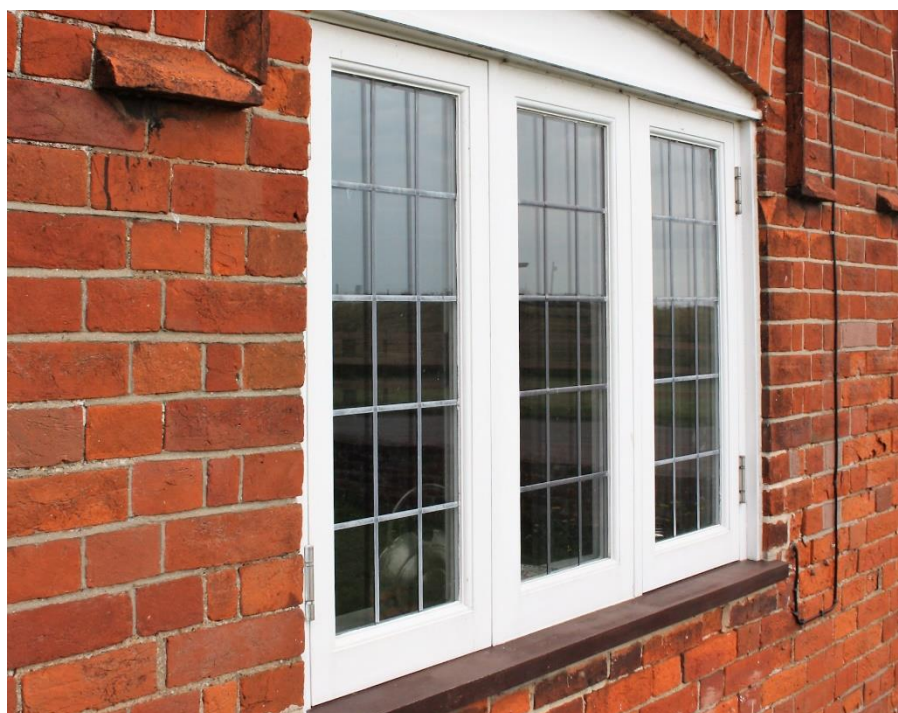
The imitation lead comes glued onto the face of this double-glazed window reflect off the inner leaf of the sealed unit, creating an appearance that is quite different to traditional lead glazing
