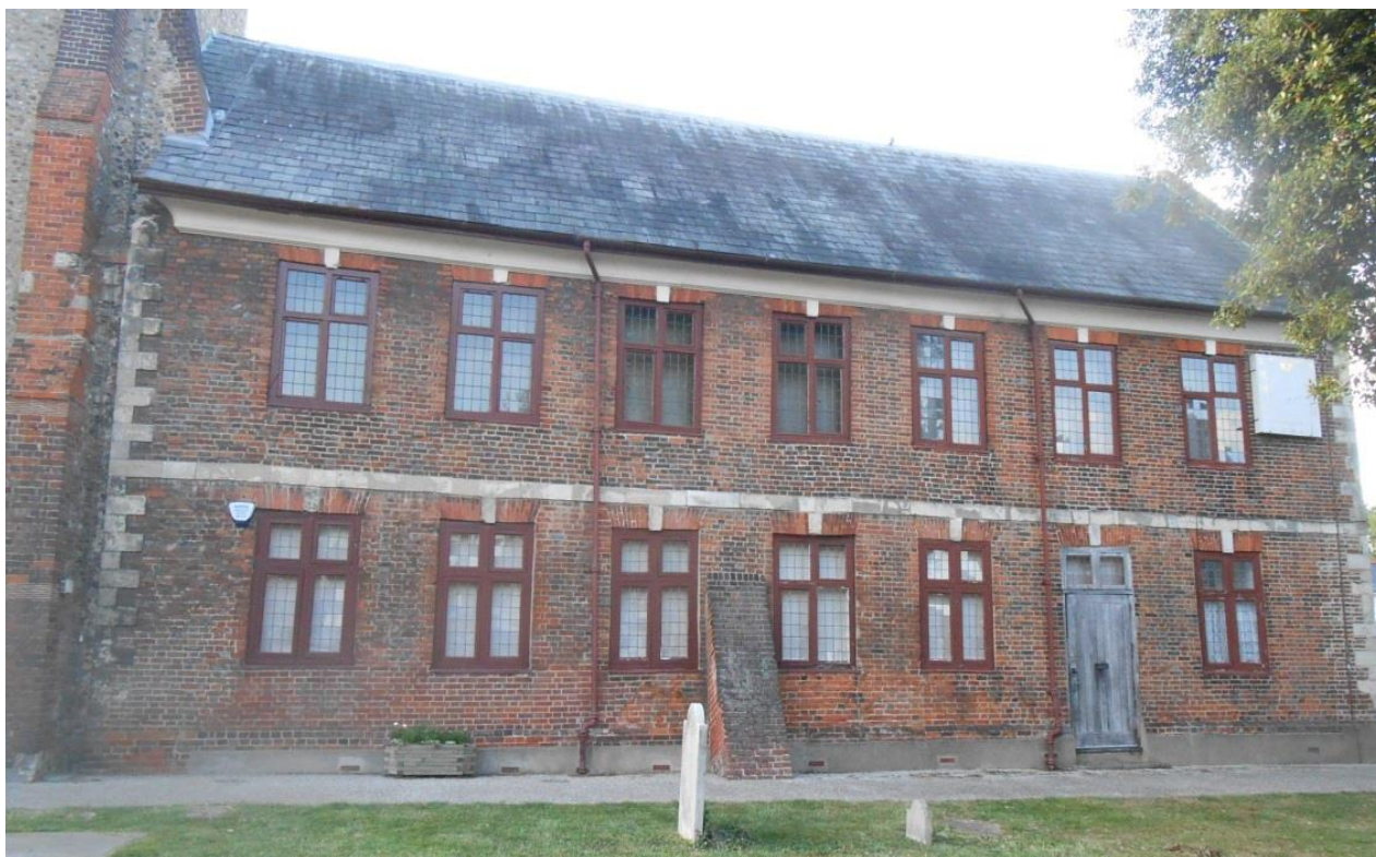
Early-20th century lead-glazed cross windows in a library of c.1699. The windows replicate the design of late-17th-century windows
