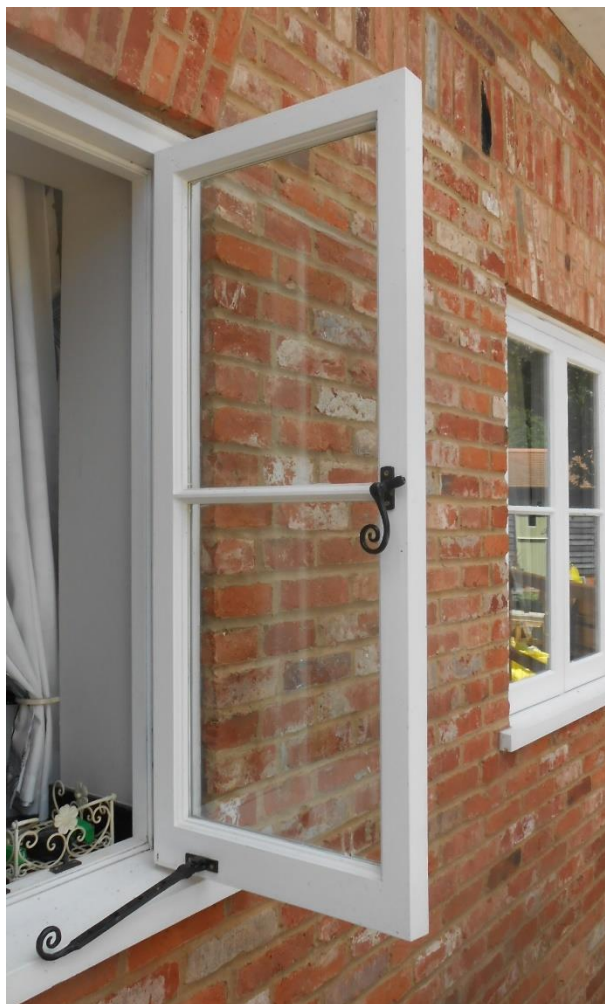
Casement windows with slim-profile double glazing, made by Kevin Gribble of Maeldune Bespoke
