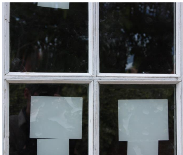
Sealed units held in place by timber fillets
