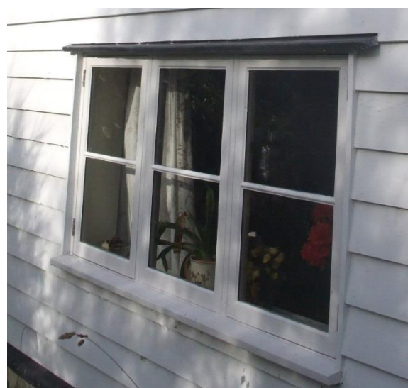
Casement window with slim-profile double-glazed units installed in 2011
