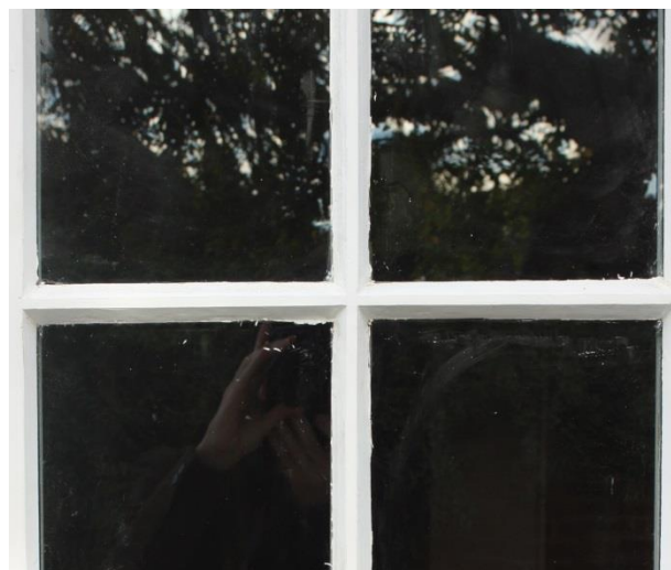
Sealed units held in place by Butyl putty
