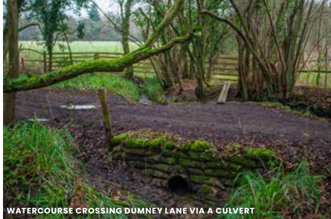
WATERCOURSE CROSSING DUMNEY LANE VIA A CULVERT
