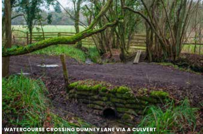
WATERCOURSE CROSSING DUMNEY LANE VIA A CULVERT
