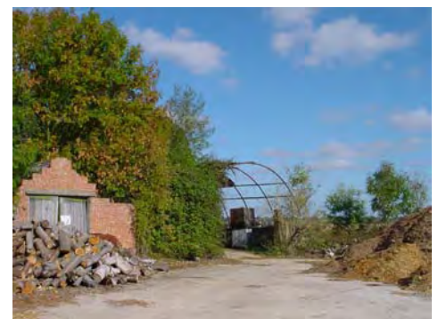
Derelict buildings near North End Place
