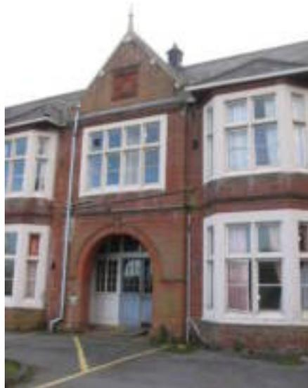
Originally a workhouse designed by William Thorold, 1837-38. Mostly destroyed by fire in 1886. Infirmary retained, red brick, gabled slate roof, small paned sash windows, some alterations to fenestration.
