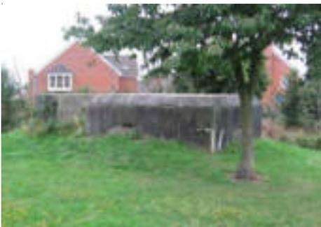
Pillbox, c.1940. Rectangular form with three small gun apertures. Entrance now blocked. Concrete blast wall to the SW, with a single gun aperture. Positioned 50yds SW of the former GHQ anti tank ditch.
