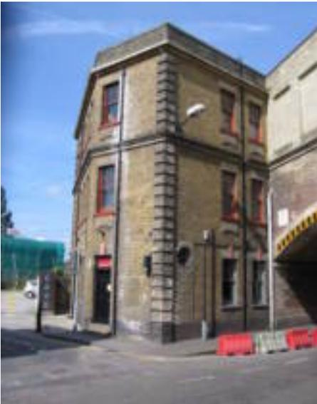
windows, with gauged brick arches incorporating a key stone on ground floor, stone cills, stone cornice and moulded brick string course, brick quoins to corner. Signal box, 1856, gault and yellow brick, timber cladding to top section, two brick arches abutting the viaduct.
