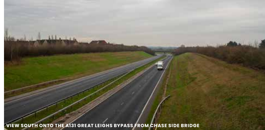
VIEW SOUTH ONTO THE A131 GREAT LEIGHS BYPASS FROM CHASE SIDE BRIDGE
