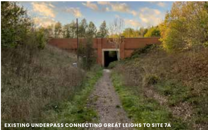
EXISTING UNDERPASS CONNECTING GREAT LEIGHS TO SITE 7A
