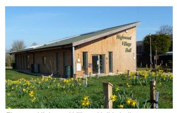
Figure x: Highwood Village Hall is built to Passivhaus principles with excellent thermal performance and airtightness. The triple glazed windows are oriented to the south, west and east to maximise natural solar gain and the roof overhang provides shading. Solar panels and an air source heat pump provide electricity and heating.
