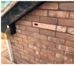
Figure X: Swift bricks should be installed high up in gable ends or directly under eaves
