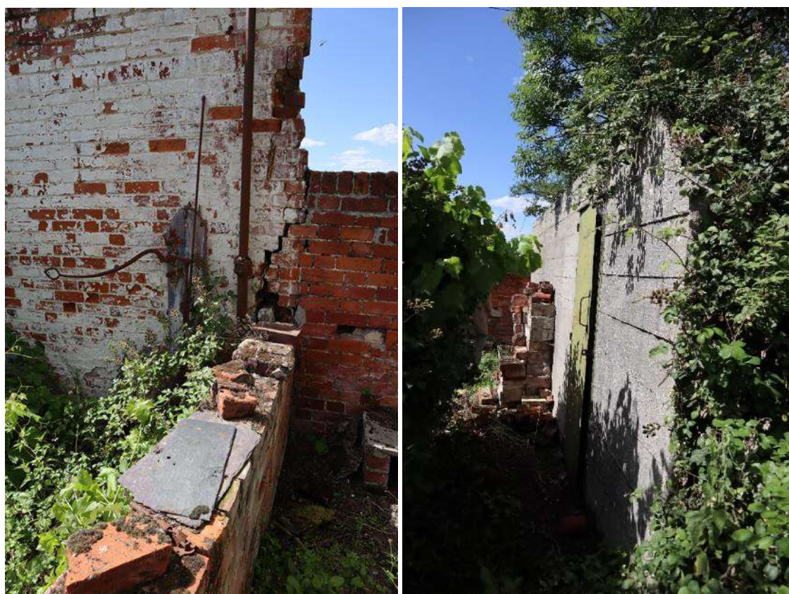
Figure 31 – lime washed rear wall of the glass house, the internal wall, with the lowered viewing section and the pillbox
