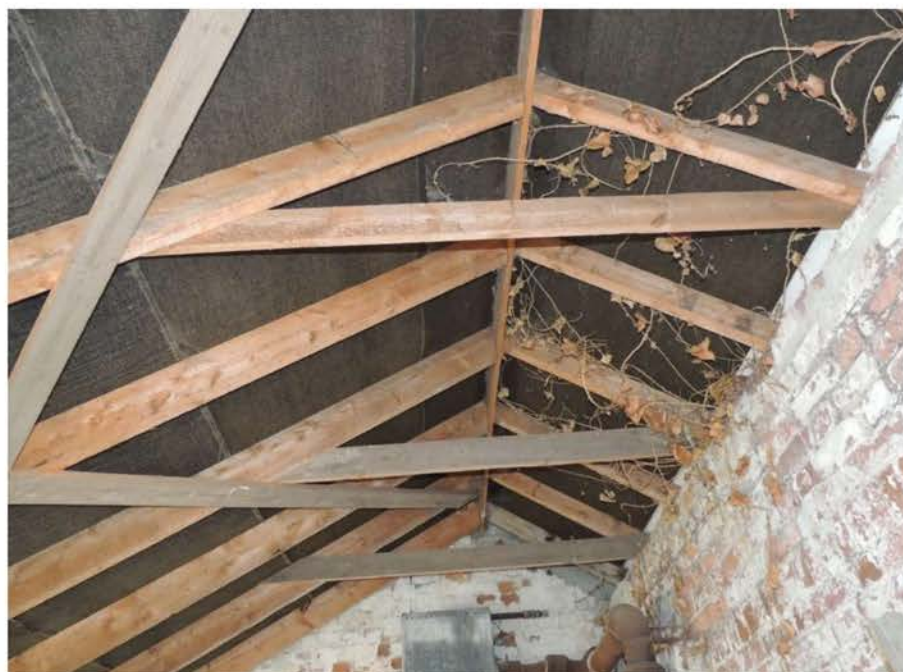
Photo 6: Insulation is to be placed between the rafters. The roofing felt is unaffected
