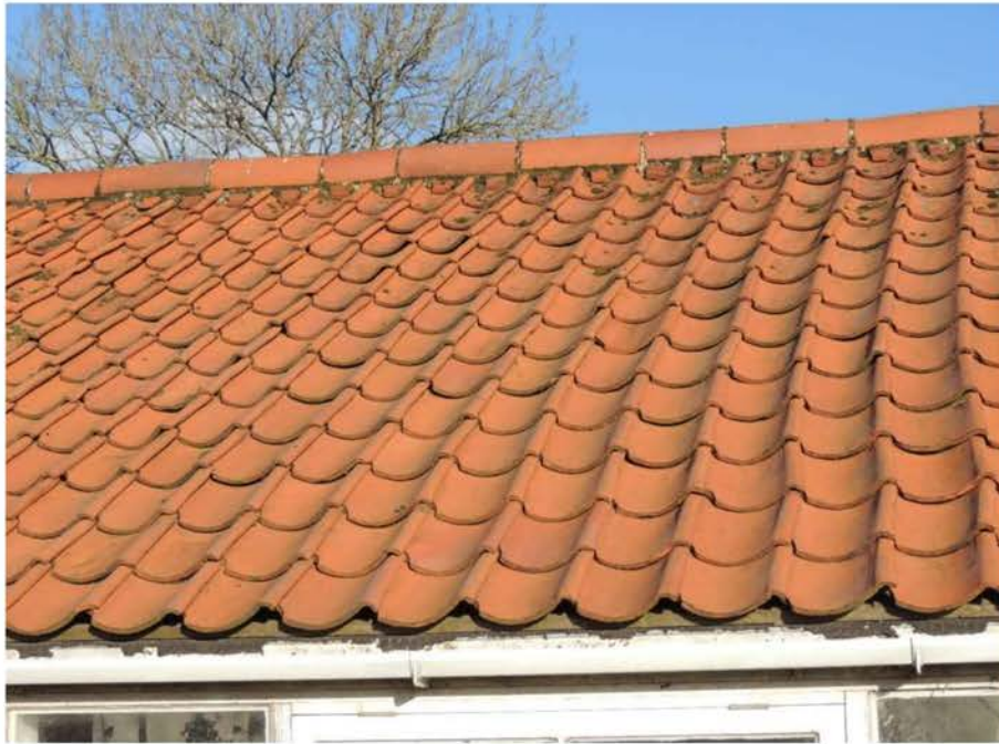
Photo 7: Note tight seal to pantiles
