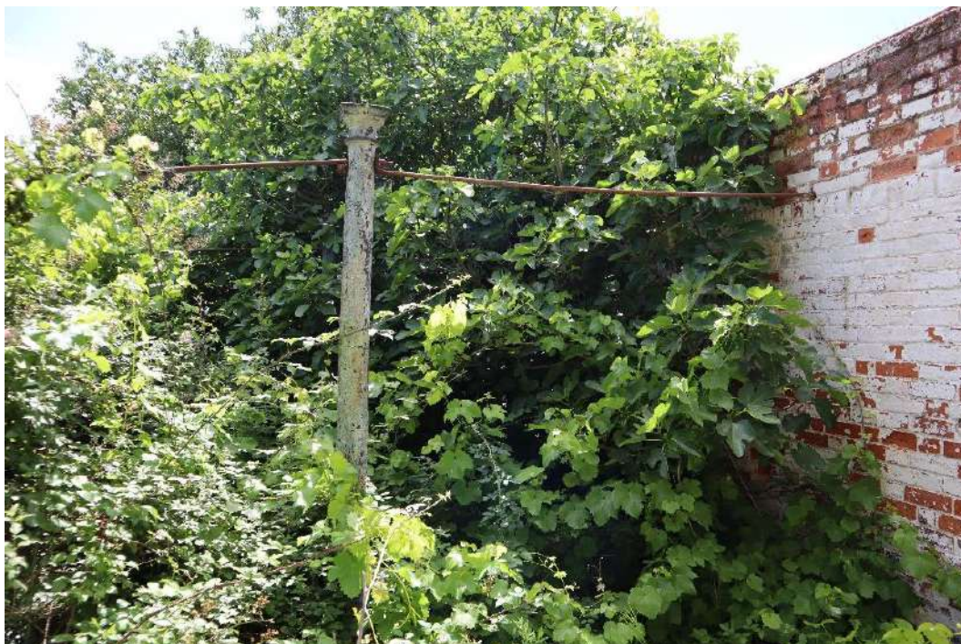
Figure 14 – delicate support posts and ties, with limewashed rear wall
