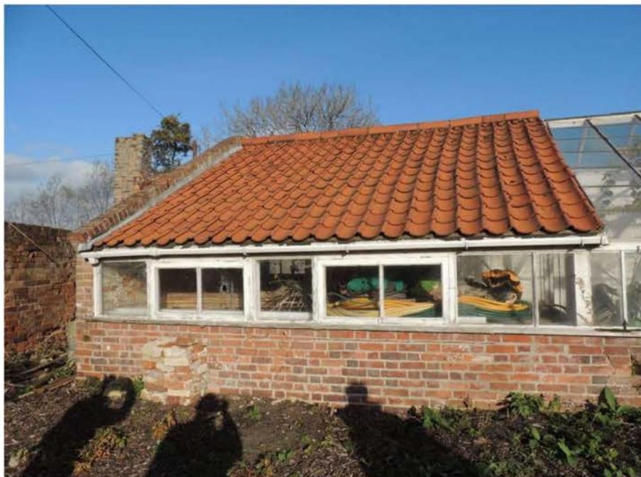
Photo 1: South-western elevation. The proposal is to insulate the roof on the inside of the building. The existing pantiles and roofing felt are unaffected by the proposal
