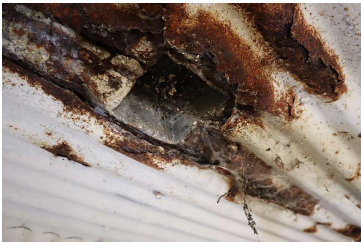
Figure 46 – limited damage due to water ingress due to formed square opening in roof
