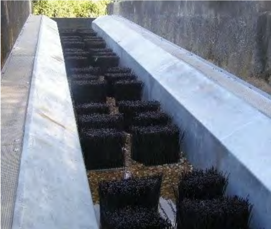
Image of empty canoe chute showing fish pass built in
