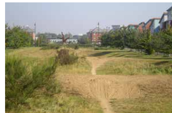
SuDS infiltration basins have been integrated with highways at Ravenswood in Ipswich. The scheme is estimated to have saved over £600,000 in the long term (Ipswich Borough Council, 2011)
