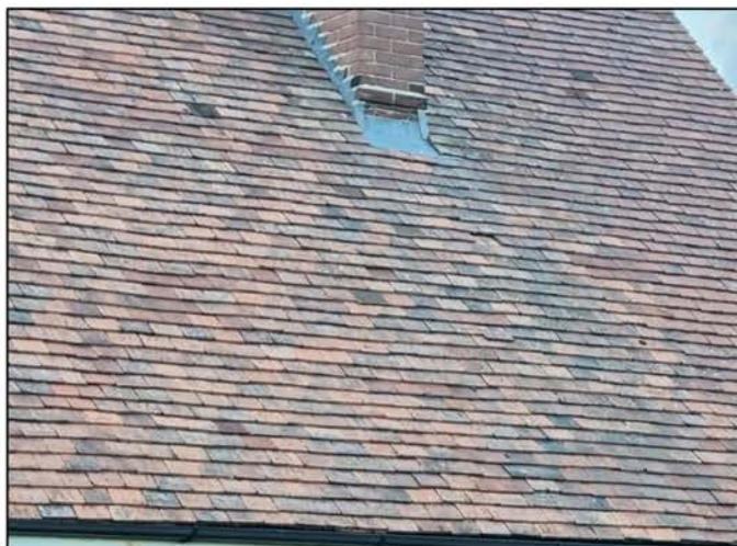
c) Missing roof tile on southern aspect
