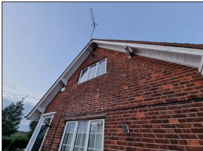
b) Western gable – intact, well-sealed
