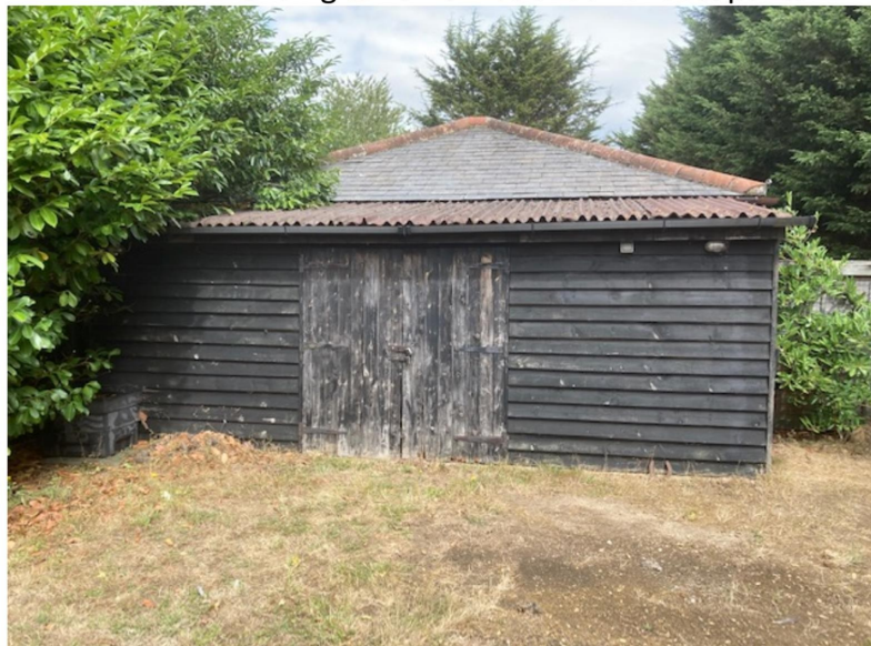
Photo 2 - Building to remain as shed for occupants
