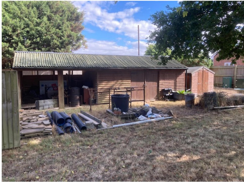
Photo 1 - Buildings to be demolished
