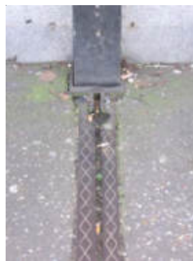
Figure 35 Cast iron rainwater gully
