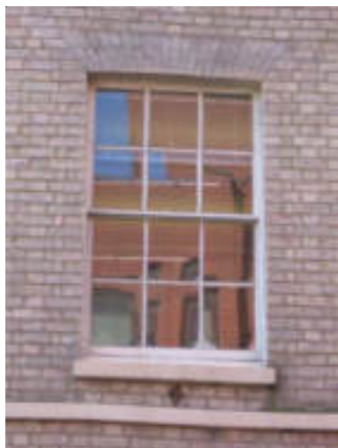
Figure 23 Small panel, finely detailed early C19 sash set in a deep reveal
