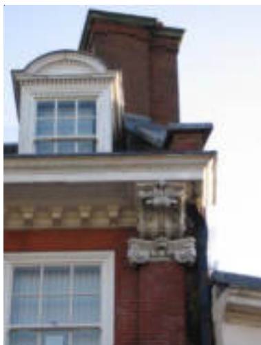
Figure 22 Small panel early C20 sash window
