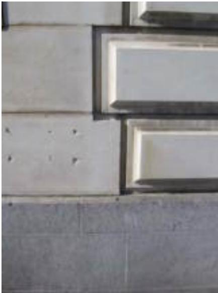
Figure 18 County Hall stonework detail, granite plinth with Portland stone ashlar cladding
