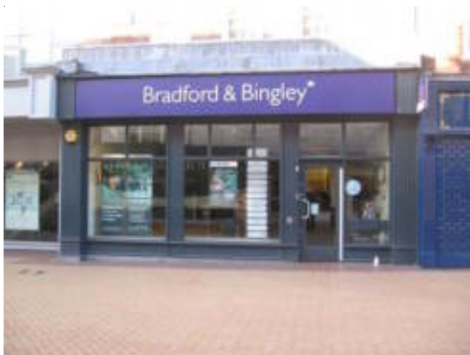
Figure 27 Modern painted timber shopfront with stall riser and pillasters
