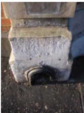
Figure 37 Cast iron bootsop
