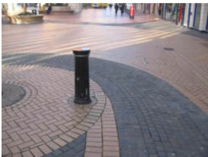
Figure 34 High street paving with clay blocks and stone setts
