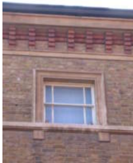
Figure 19 Brickwork detail, with different brick and string course details
