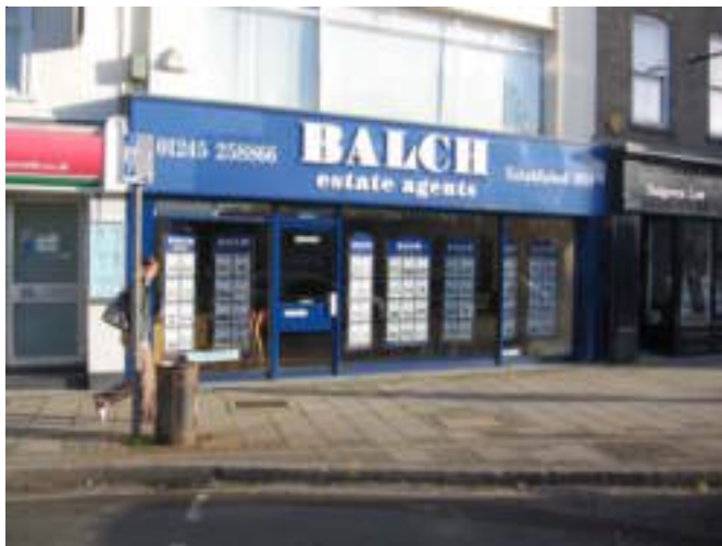
Figure 29 Inappropriate plate glass shopfront with aluminium frame and deep plastic fascia
