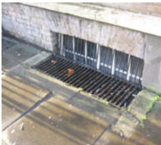
Figure 36 Cast iron basement lightwell grill
