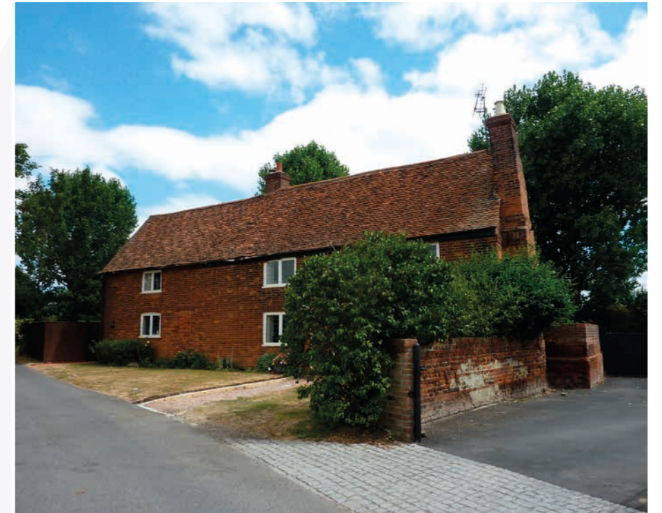
Listed Peverel’s Farmhouse
