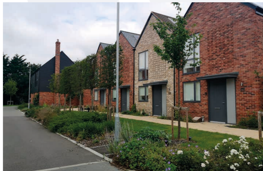
Existing Channels Complex
