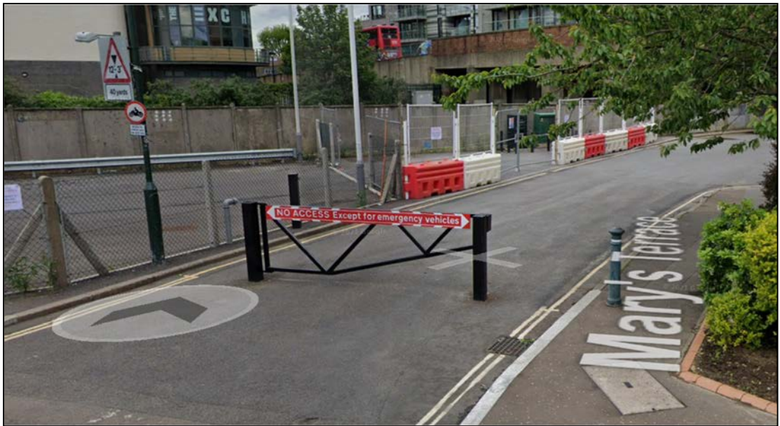
Figure 5: Example of Highways Gate
