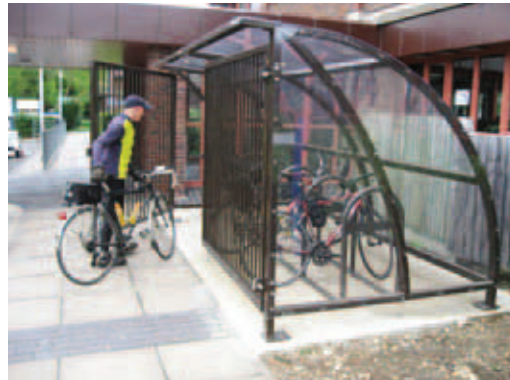
Covered shelter secured with lockable gates
