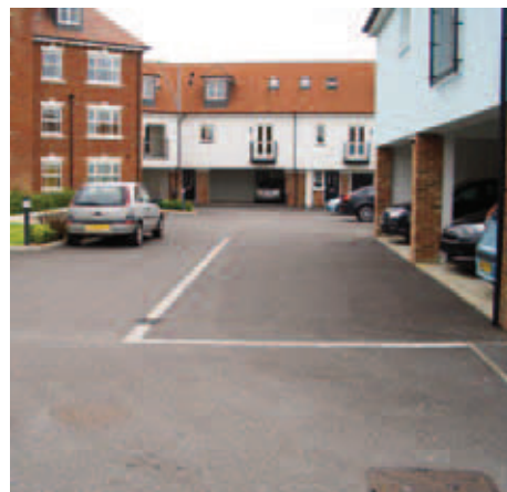
Visible undercroft parking
