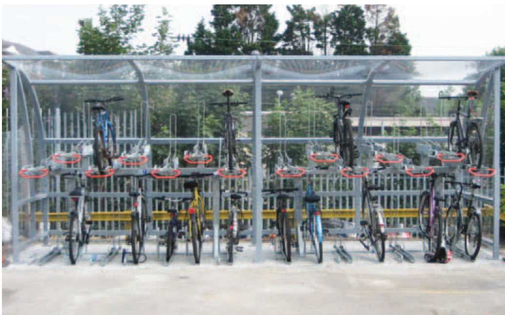
Two tier racks within covered cycle shelter
