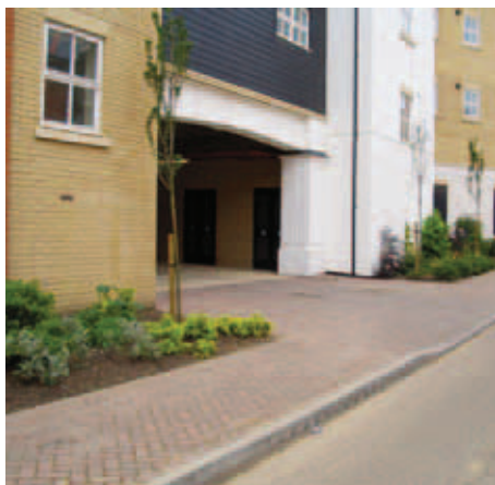
Undercroft secure parking (gated entry).
