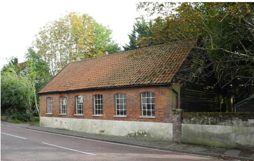
Fig. 35 Rectory Hall. The use of cement render has disfigured the building and the boundary wall, and exacerbated the damp problem it was meant to cure
