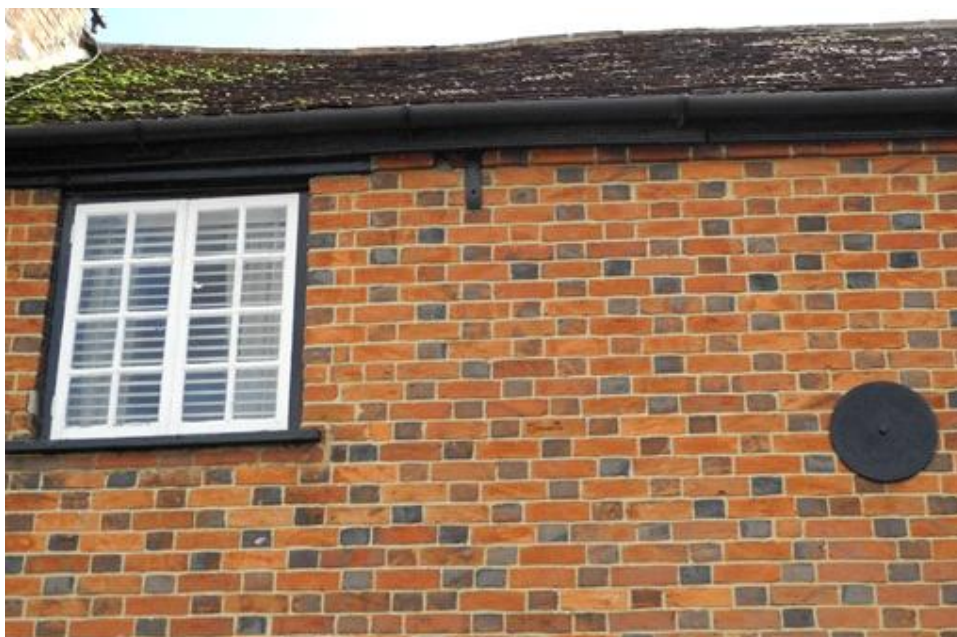
Fig. 8 18th century brickwork with regular use of flared headers. Note the diagonal skintlings
