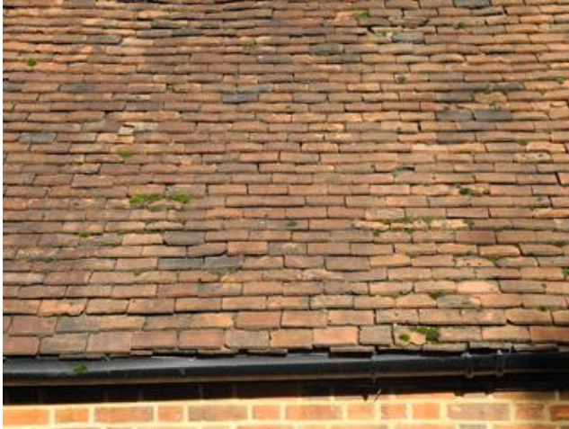
Fig. 9 The irregularity of handmade clay pegtiles gives life and character to roofs
