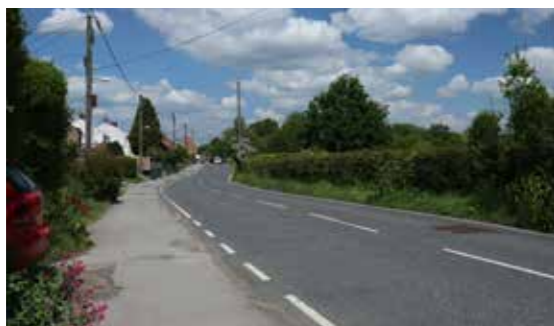
4. Molrams Lane looking north alongside Site 3c boundary.
