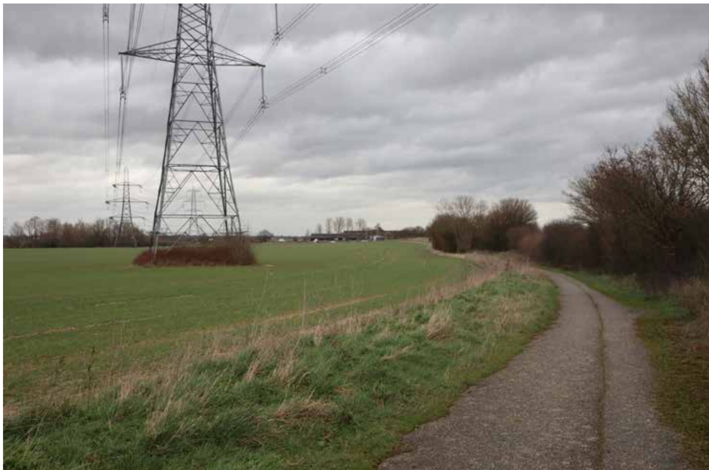
Northern boundary to NCN R1. Note extent of mature hedgerow, which forms a barrier to connectivity except at the point of the footpath. There is also a level change at the boundary, NCN R1 (14) is set slightly below the field level and there is a ditch.
