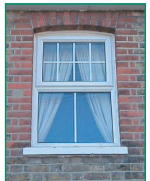
Replacement window, keeping the original opening and reveal
