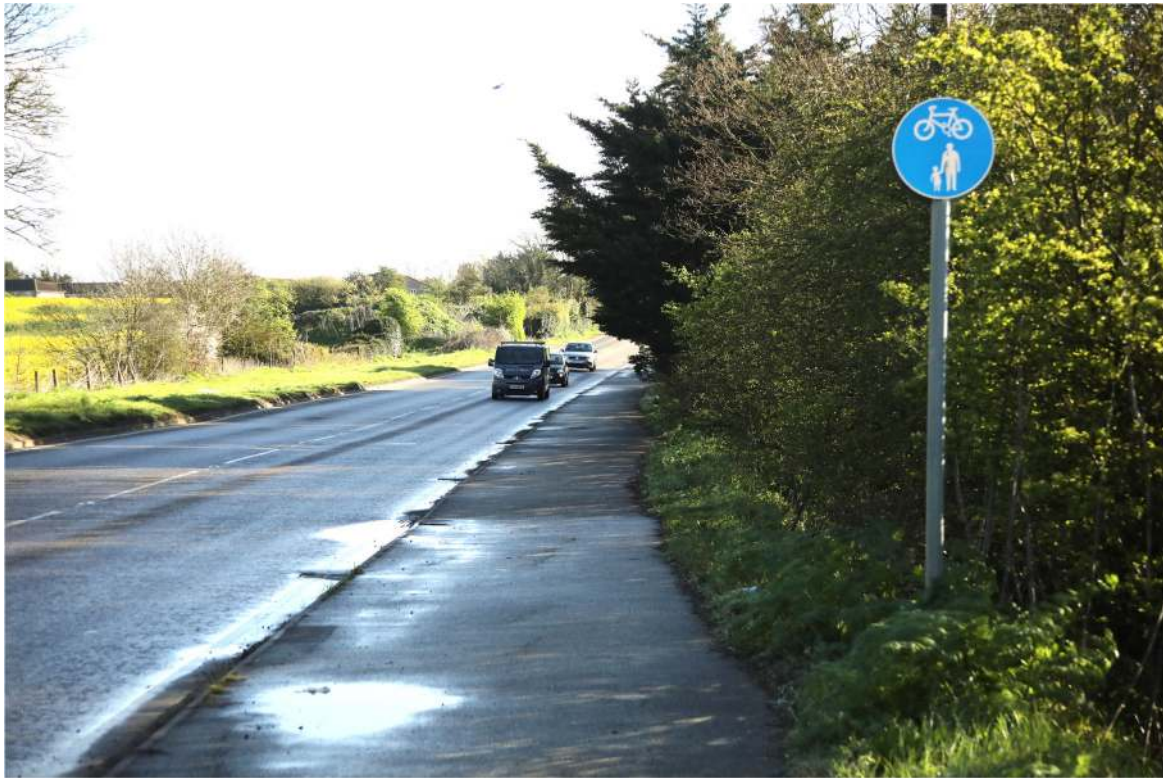
Figure 3.23 Shared use cycle path along Main Road
