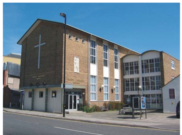
Trinity Methodist Church, 1961. Socially and architecturally important
