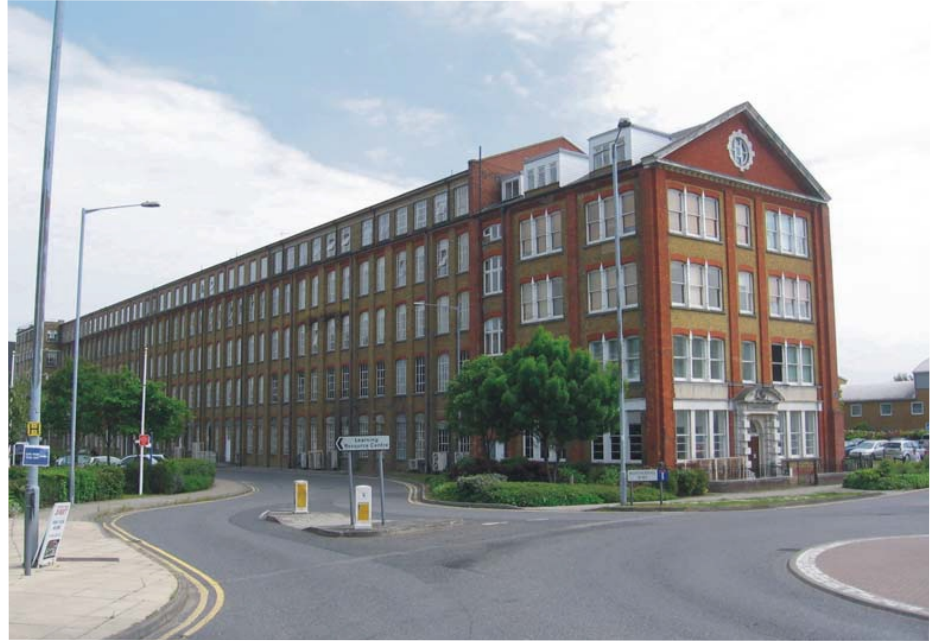
Globe House, New Street. Built as 'Hoffmanns' ballbearing factory 1897. An important remnant of Chelmsford's industrial heritage and a powerful landmark.
