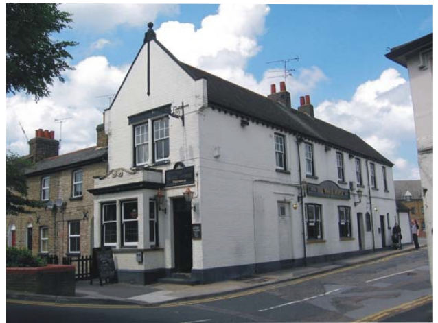
White Horse Public House, one of a number of mid c19 pubs of townscape, historic and architectural interest
