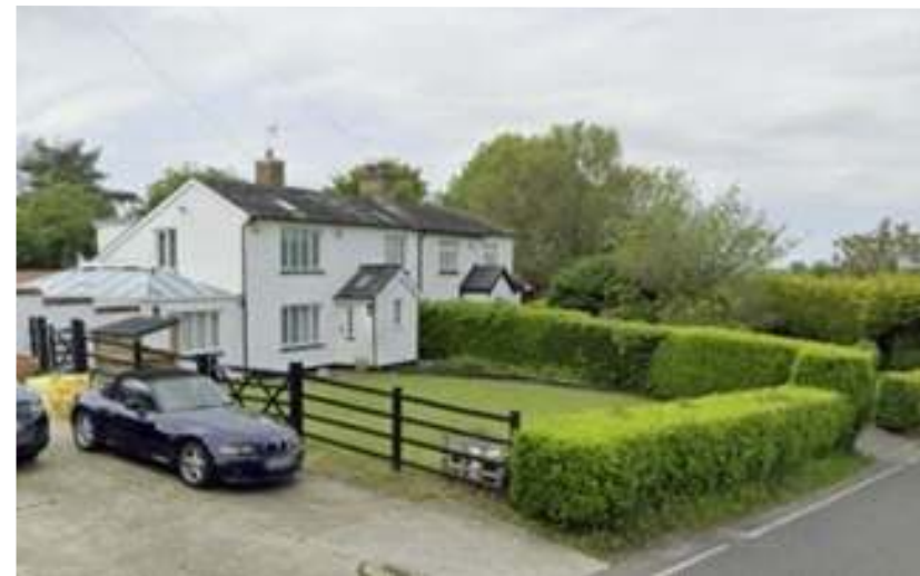
Fig.24 Hill Cottage and Florence Cottage Mid-nineteenth century.
