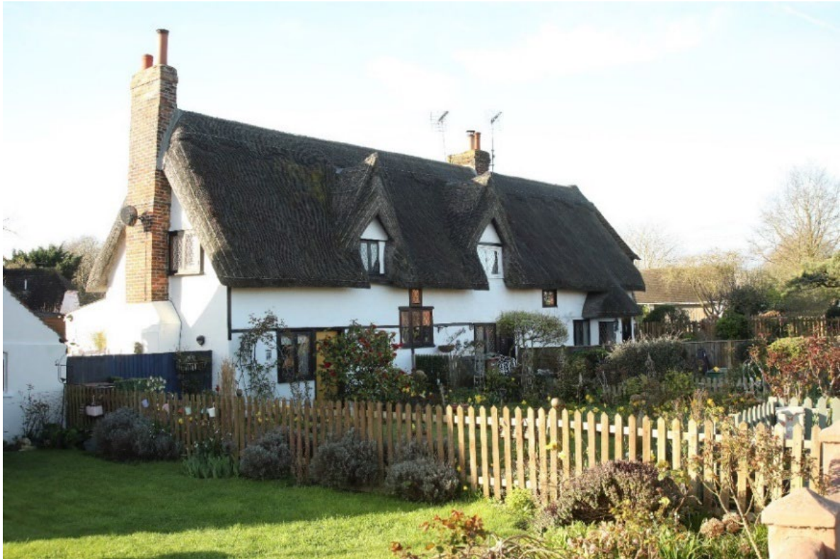
Figure 3.29 Maltings Cottages, Main Road
