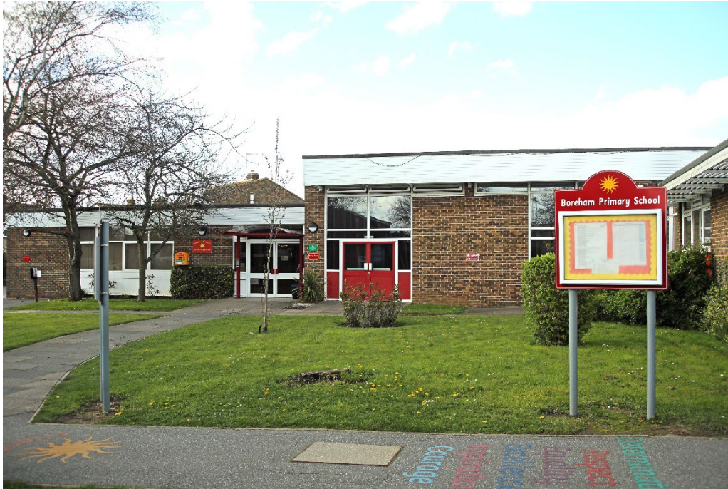
Figure 3.20 Boreham Primary School
