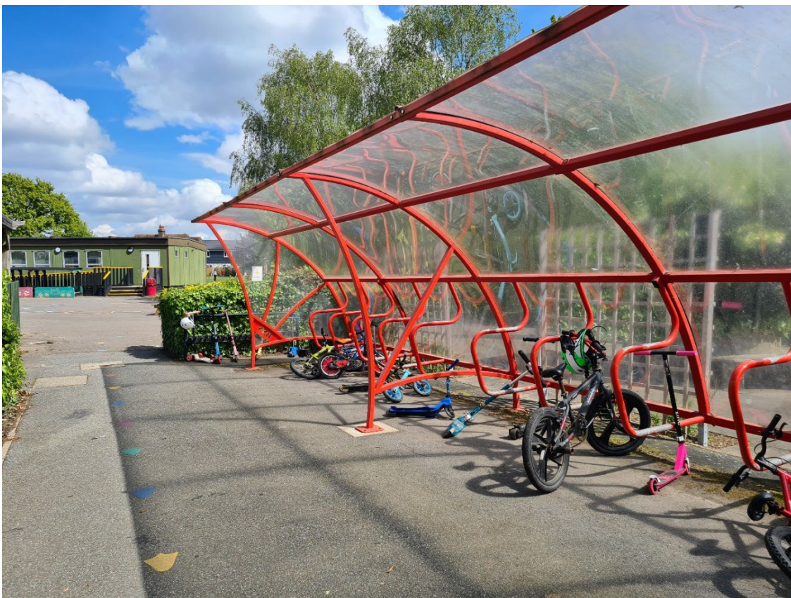
Figure 5.11 Boreham Primary School cycle and scooter storage facility
