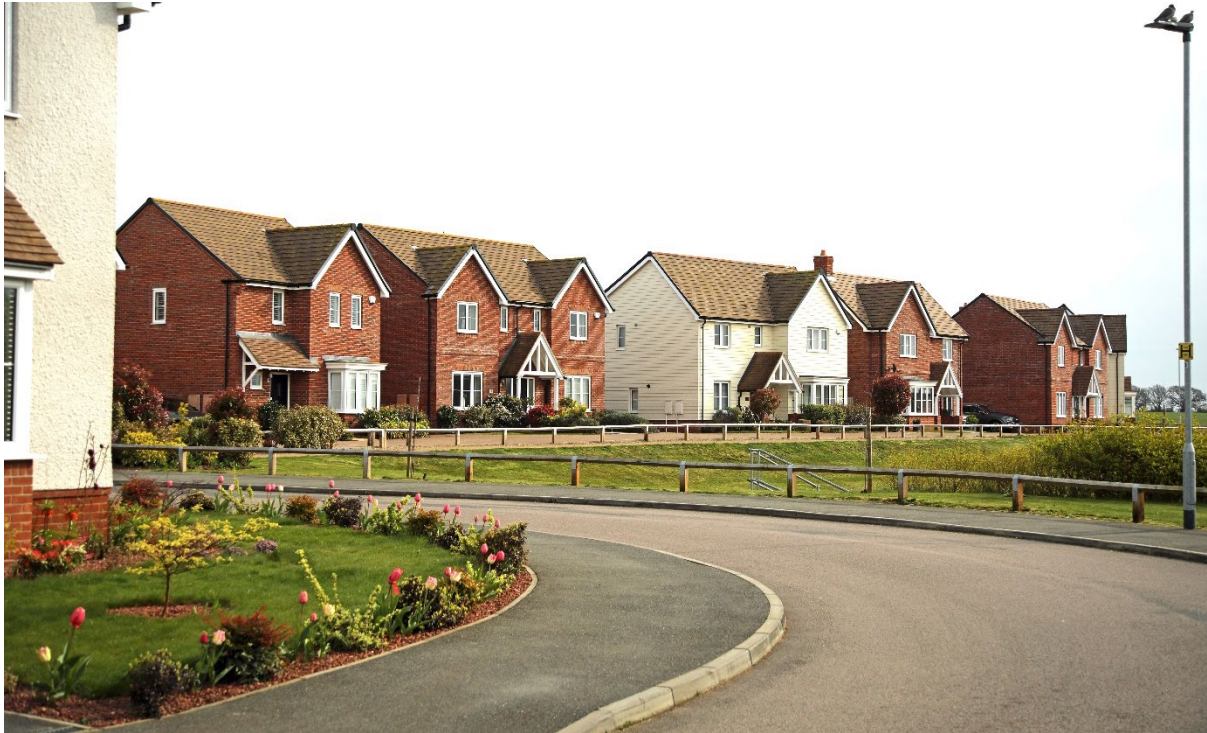
Figure 3.26 Houses in the Orchard Way development
