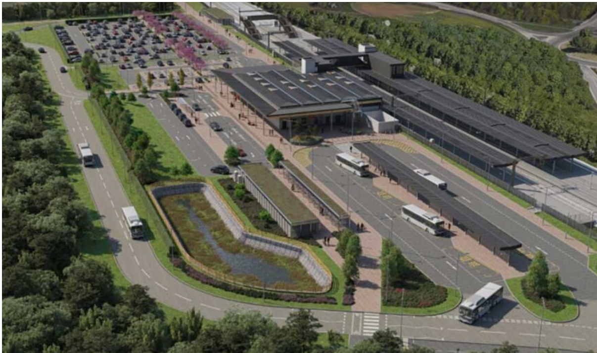
3.24 An artist's impression of the new Beaulieu Park Railway Station courtesy of Network Rail
