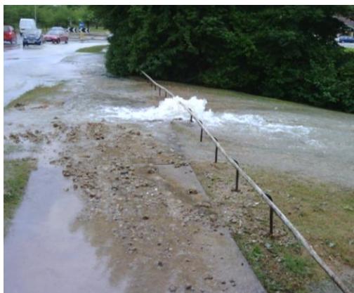
Figure 3—8 Surcharging of the sewer system within a road (left) and internally within a property (right)
