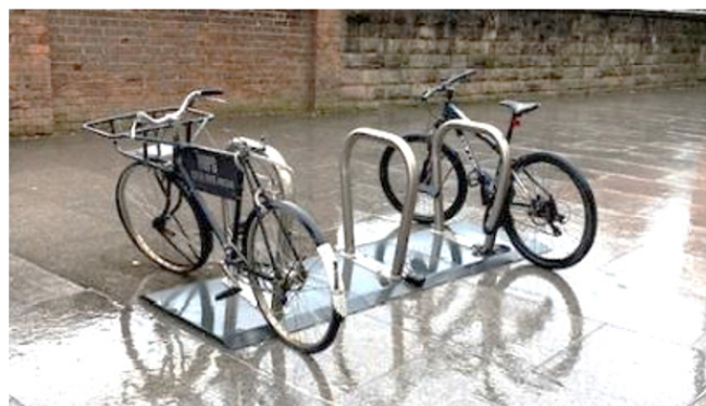
Figure 3-4: Recommended arrangements for Sheffield stand provision
