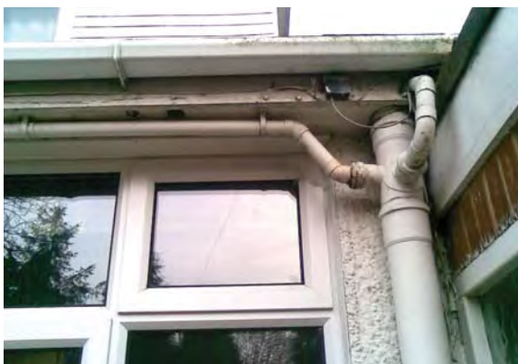
Example of exposed waste pipes
