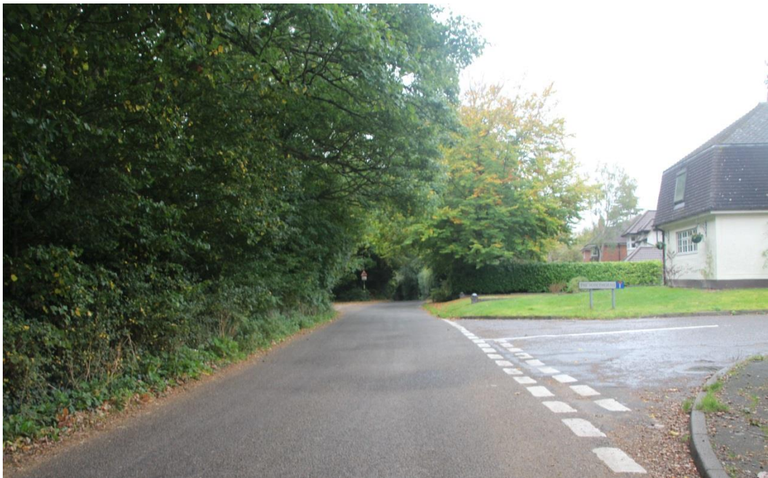
Figure 3 - New Road junction along Hyde Lane
