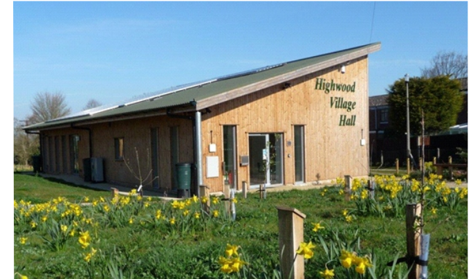
Figure x: Highwood Village Hall is built to Passivhaus principles with excellent thermal performance and airtightness. The triple glazed windows are oriented to the south, west and east to maximise natural solar gain and the roof overhang provides shading. Solar panels and an air source heat pump provide electricity and heating.
