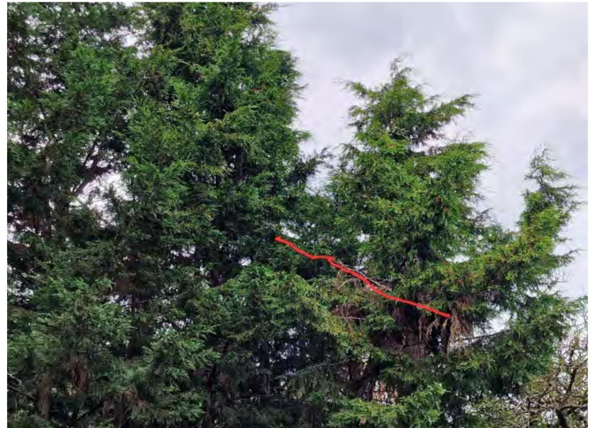
Photo 18. Leyland cypress TG11. The top of one tree has failed and is 'hung-up' over the site. This should be removed.
