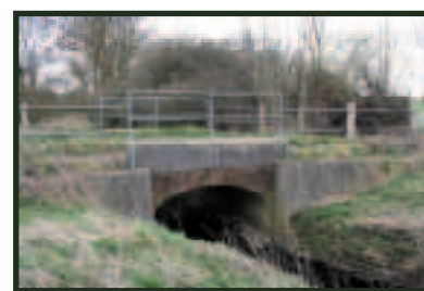
Motts Green Bridge with ugly galvanised railing and concrete
