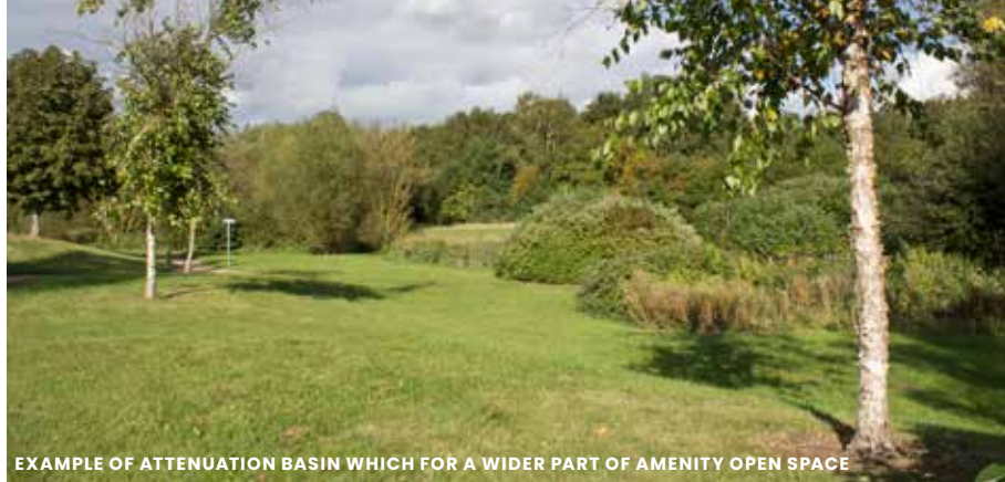
EXAMPLE OF ATTENUATION BASIN WHICH FOR A WIDER PART OF AMENITY OPEN SPACE
