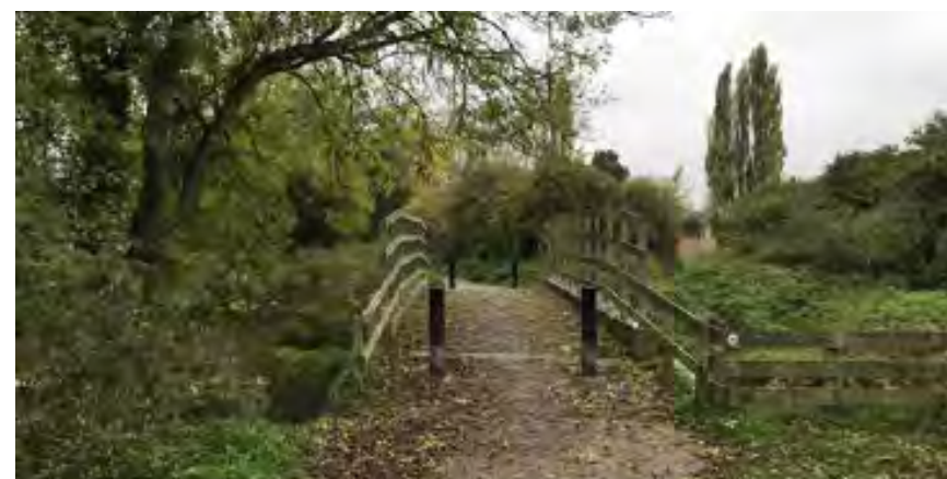
Figure 11: Footbridge over the River Can along Lawford Lane (source: AECOM)
