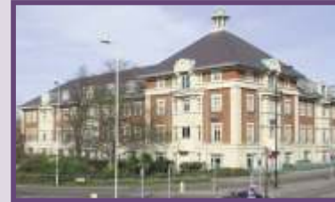
Parkview House, Victoria Road South
