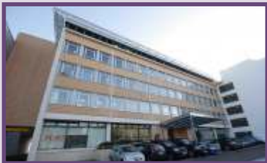
Greenwood House, New London Road
