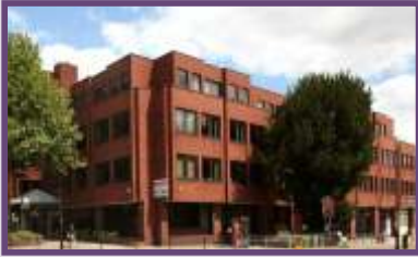
Victoria House, Victoria Road
