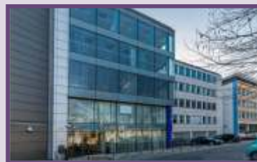
Fenton House, New London Road
